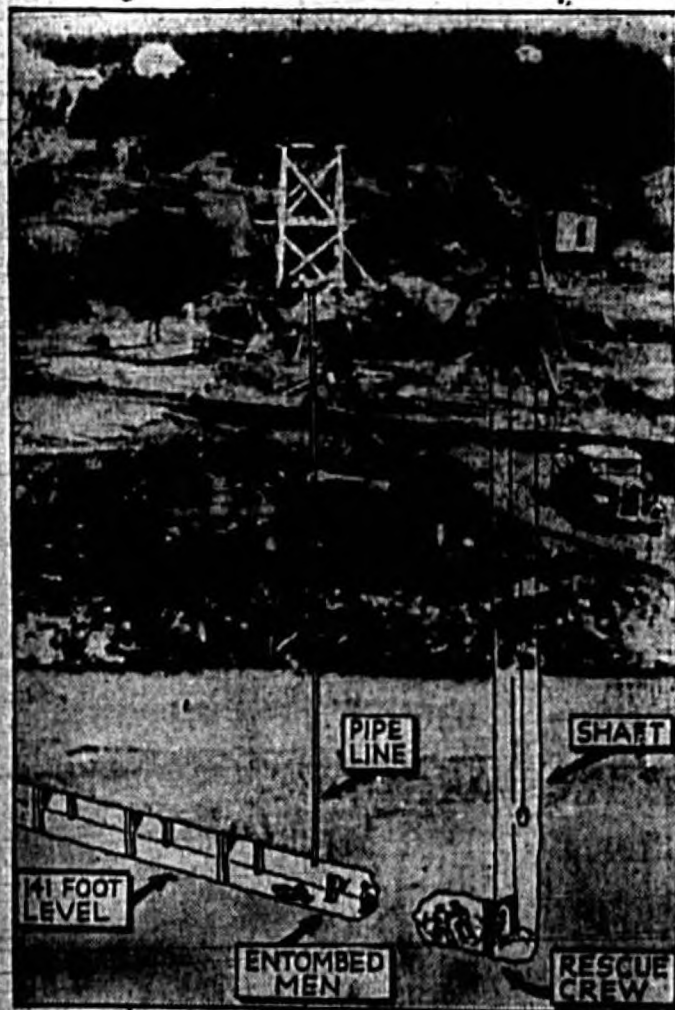
After nine days of feverish digging, rescue workers tunneled their way to Dr. D. E. Robertson and Charles A. Scadding and the body of Herman Magill who were entombed by a landslide in a gold mine at Moose River, Nova Scotia, Easter Sunday. Magill died of exposure two days before the rescue. This photo-diagram shows the location of the trapped men, the rescue shaft and the pipe line through which the communication was established with the victims. (Associated Press Photo)
