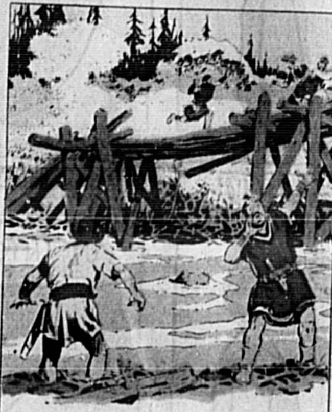
SWEPT DOWN BY THE CURRENT, THIS MASS PILES UP AGAINST THE BRIDGE PIERS, FORMING A DAM BEHIND WHICH THE RIVER RISES STEADILY.
