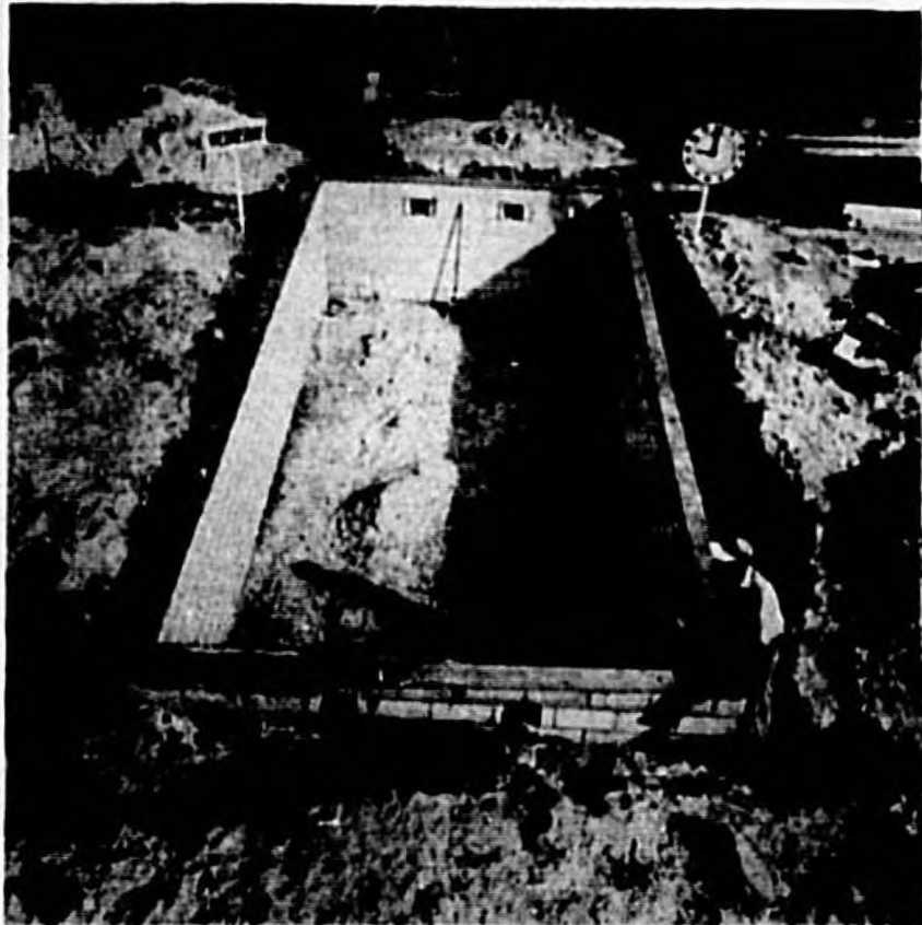
By 9 o'clock Wednesday morning, the blocks are in and the pool bottom graded. Now all that is left is to put in the plastic liner. A wood frame is shown being bolted in place to hold the liner.
