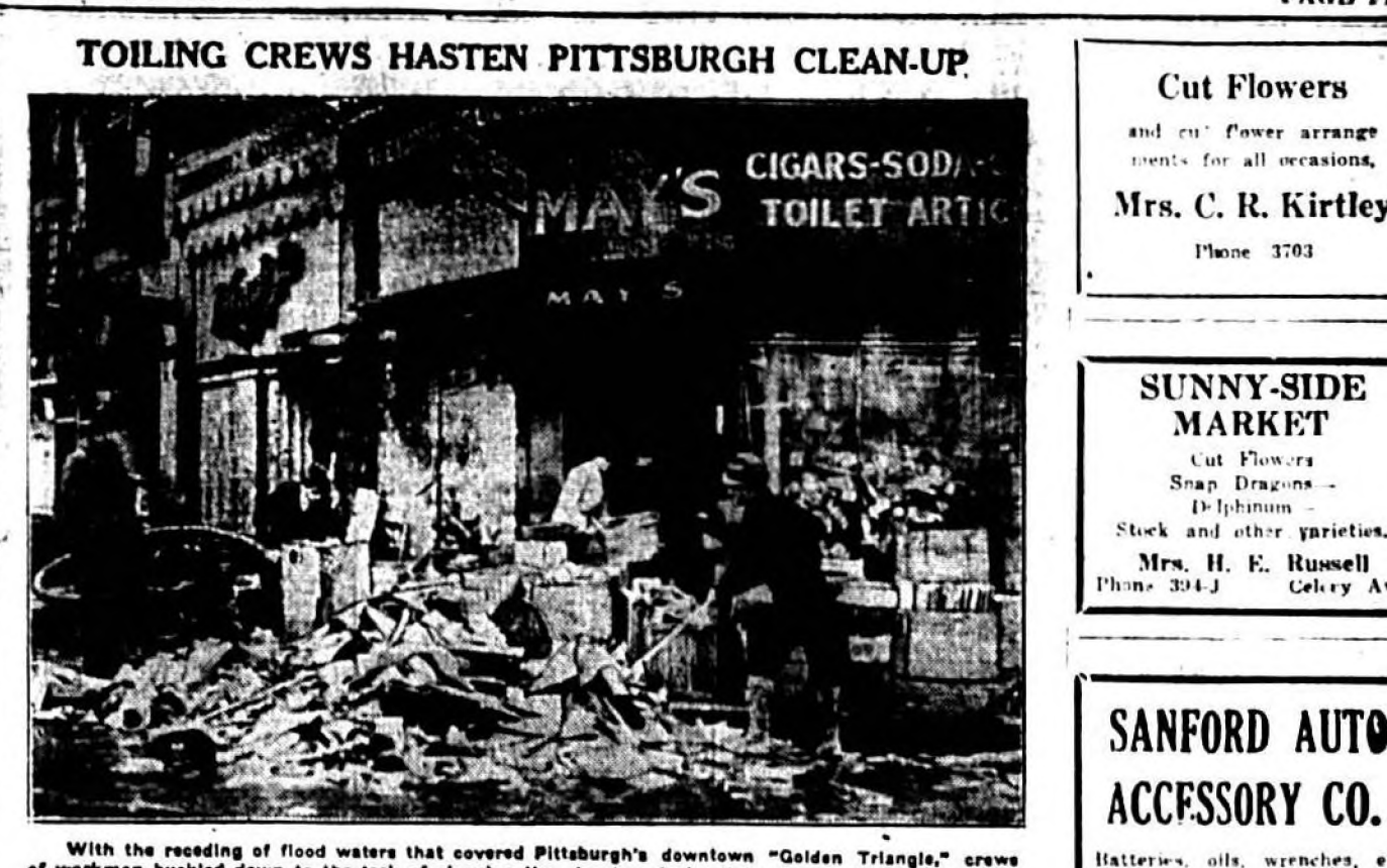
TOILING CREWS HASTEN PITTSBURGH CLEAN-UP. With the receding of flood waters that covered Pittsburgh's downtown "Golden Triangle," crews of workers hustled down to the task of cleaning the streets. A detail is shown shoveling silt and wreckage from the sidewalk. (Associated Press Photo)
