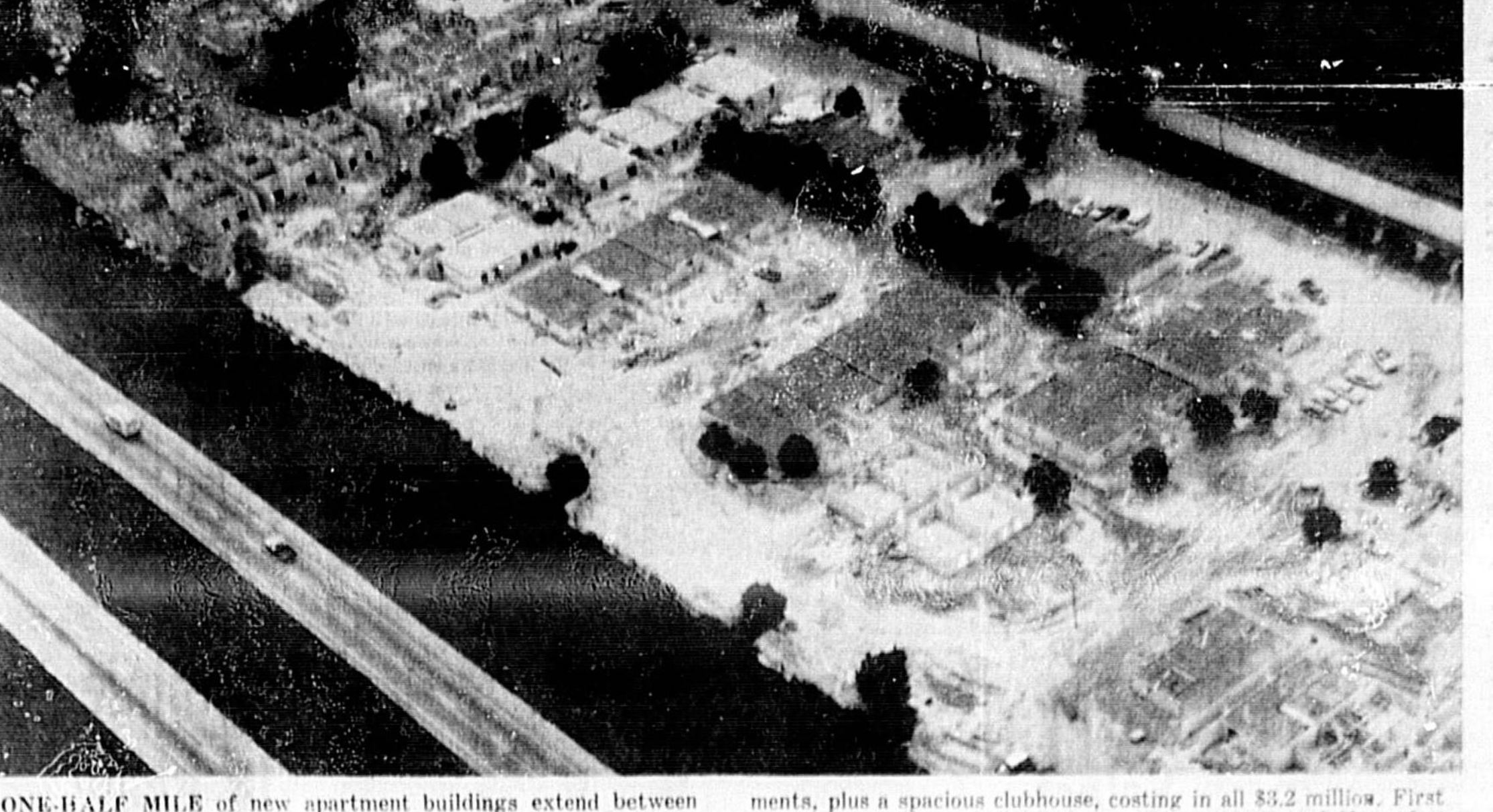
ONE-HALF MILE of new apartment buildings extend between Interstate 4 and Wynore Road south of SR 436. Demetree, First of Orlando, is currently engaged in constructing the first phase of the project. Twenty-four buildings housing 256 apartments, plus a spacious clubhouse, costing in all $3.2 million. First apartments will be available for rental at the end of November and the first phase will be completed in January. The total complex, when completed, will house 600 apartments.
