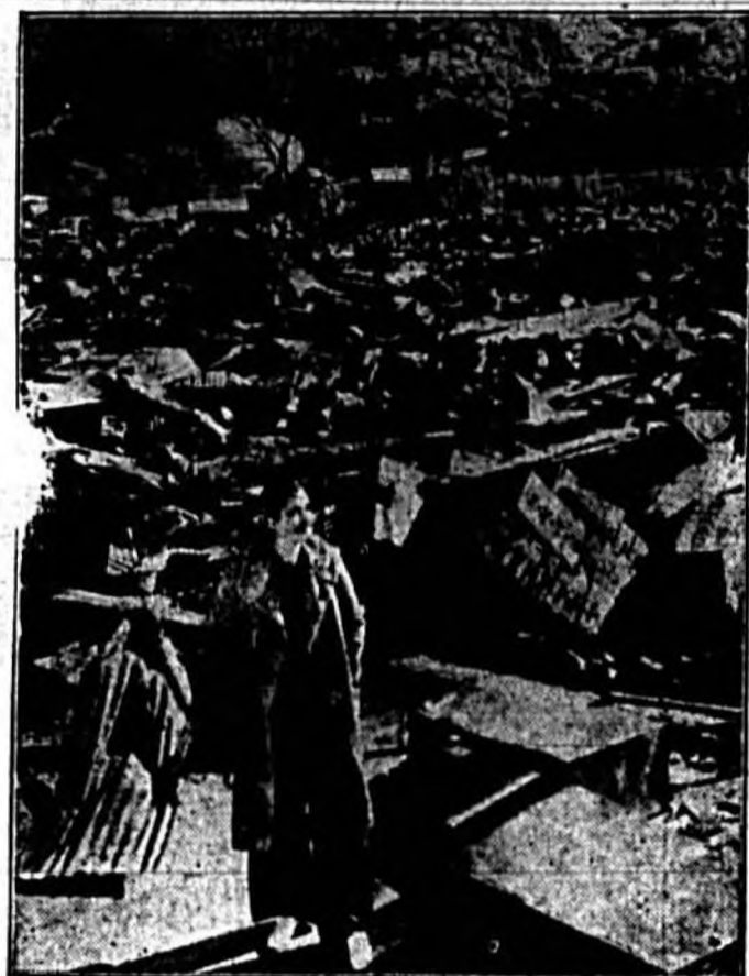
This scene of desolation—brightened only by the presence of Screen Actress Kay Francis—was left by the fire that swept half of the 80-acre movie picture studio of Warner Brothers—First National at Burbank, Calif. Estimates of the damage ranged from $200,000 to $300,000. (Associated Press Photo)
