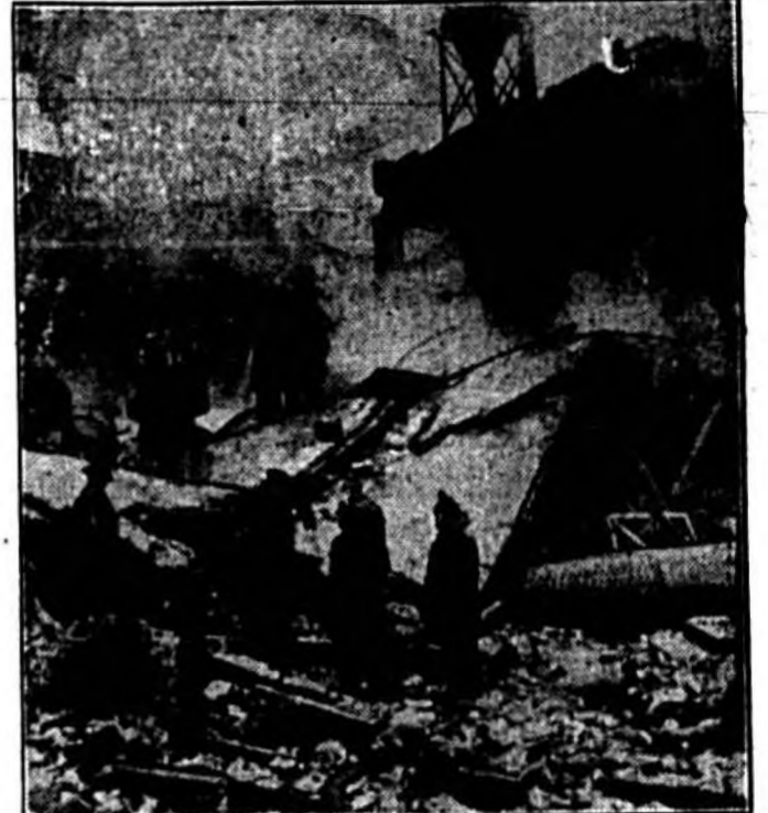
Two workmen were killed and half a dozen persons were injured seriously by an explosion that demolished the hydrogen plant of Swift and company in the Chicago stockyards. Firemen are shown searching the smoking ruins for victims. (Associated Press Photo)
