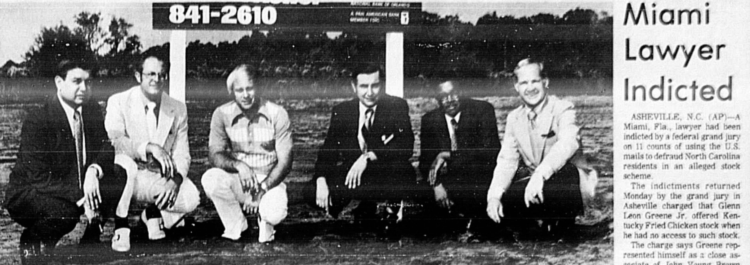
850,000 PLANT CONSTRUCTION under way in Seminole — Ground-breaking ceremonies marked beginning of Concrete Structural Systems of Florida, Inc.'s new structural room unit plant, being built on Seminole County Port Authority property. Citizens National Bank of Orlando is providing financing. At left, Mayor... (right) Jim Johnson, executive vice president of CSSI, Tom Binford and Sid Vihlen, Port Authority members; Chuck Keller, Citizens National Bank of Orlando; Ed Blackshear and Jim Ryan, Port Authority members.
