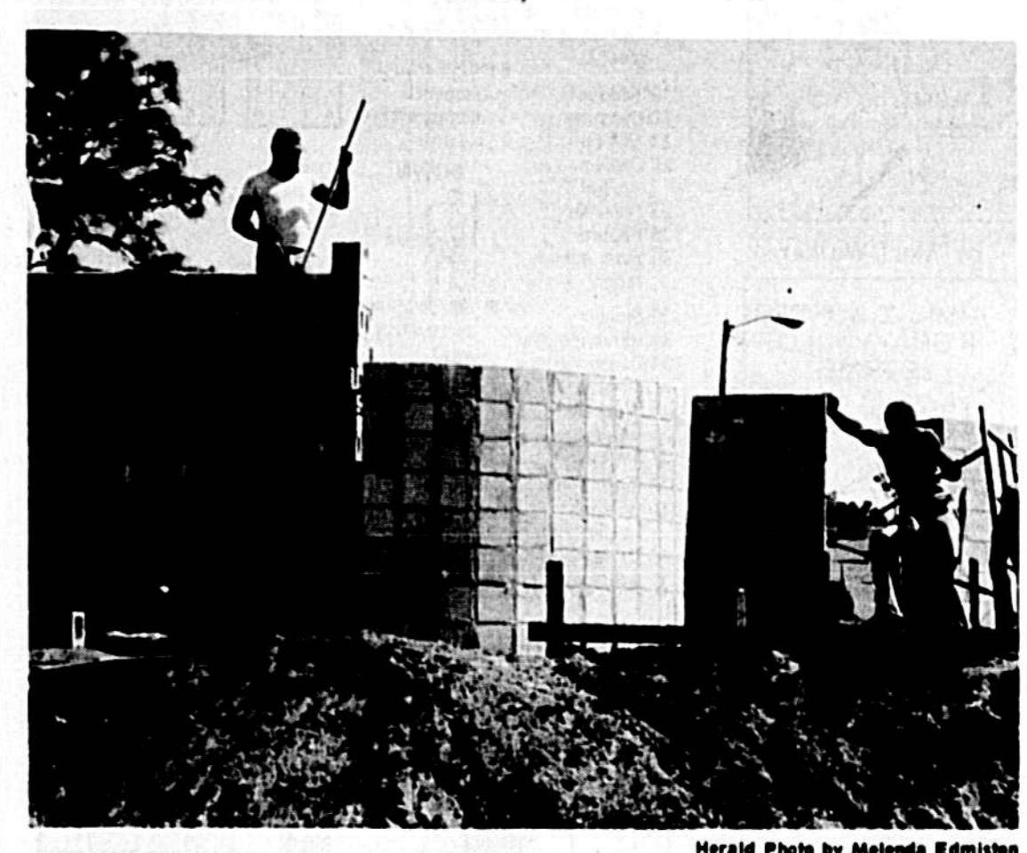
Walls are going up on the new church building being constructed by Walker & Co. general contractor for St. Augustine Catholic Church on Sunset Drive, Casselberry. The $364,000 structure will be in contemporary style.
