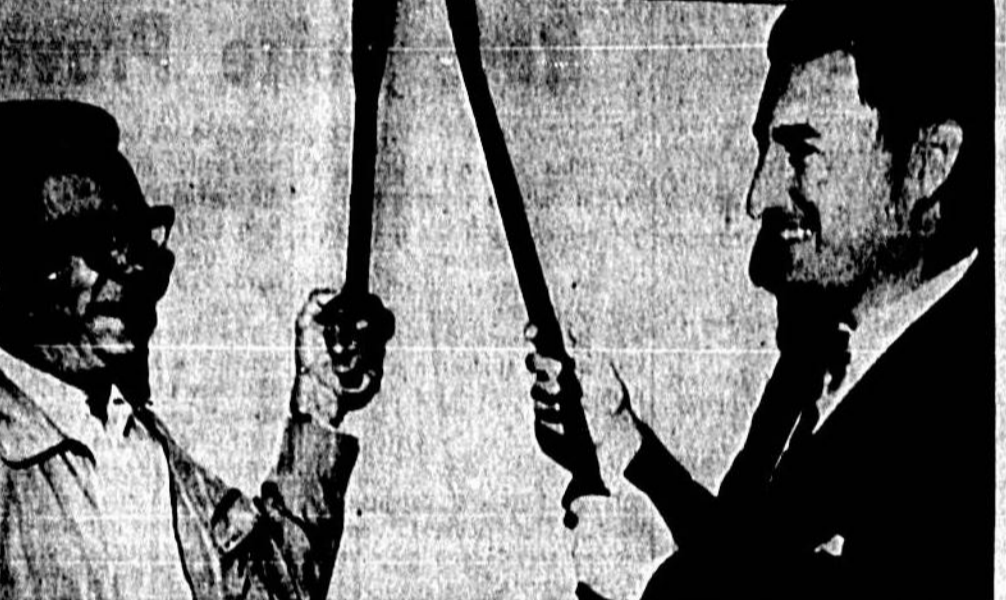
SANFORD ATLANTIC BANK expansion program kicked-off this morning. Shown above is assistant vice president DeWitt Matthews (right) and Contractor Leroy Robb with crewmembers getting the project underway.
