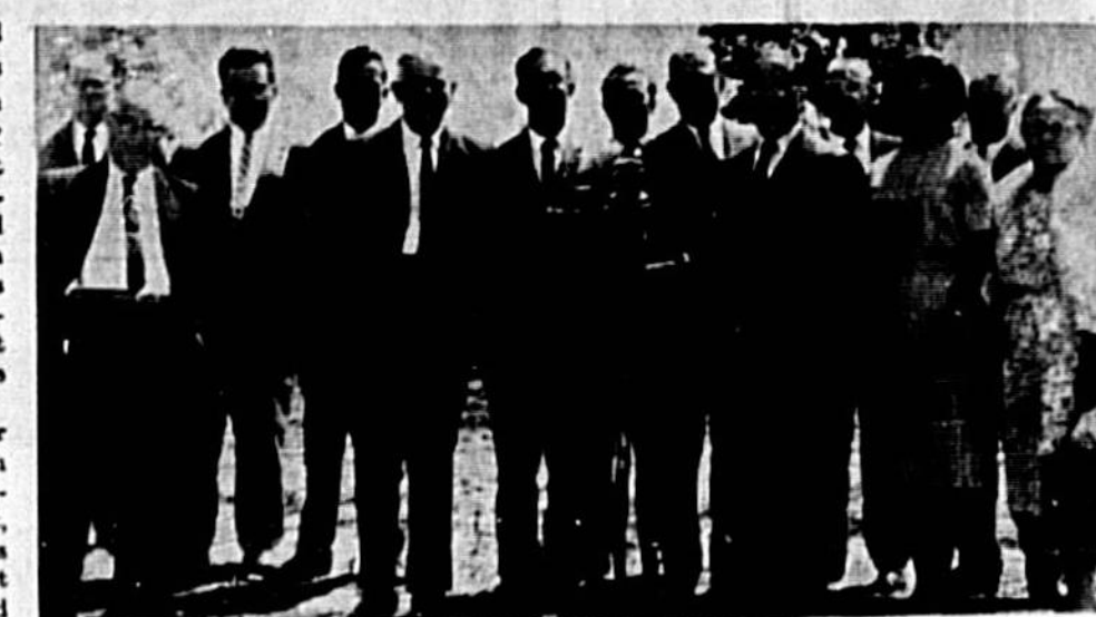
CHURCH OF GOD has broken ground for its new building at the corner of Holly Avenue and 22nd Street.
