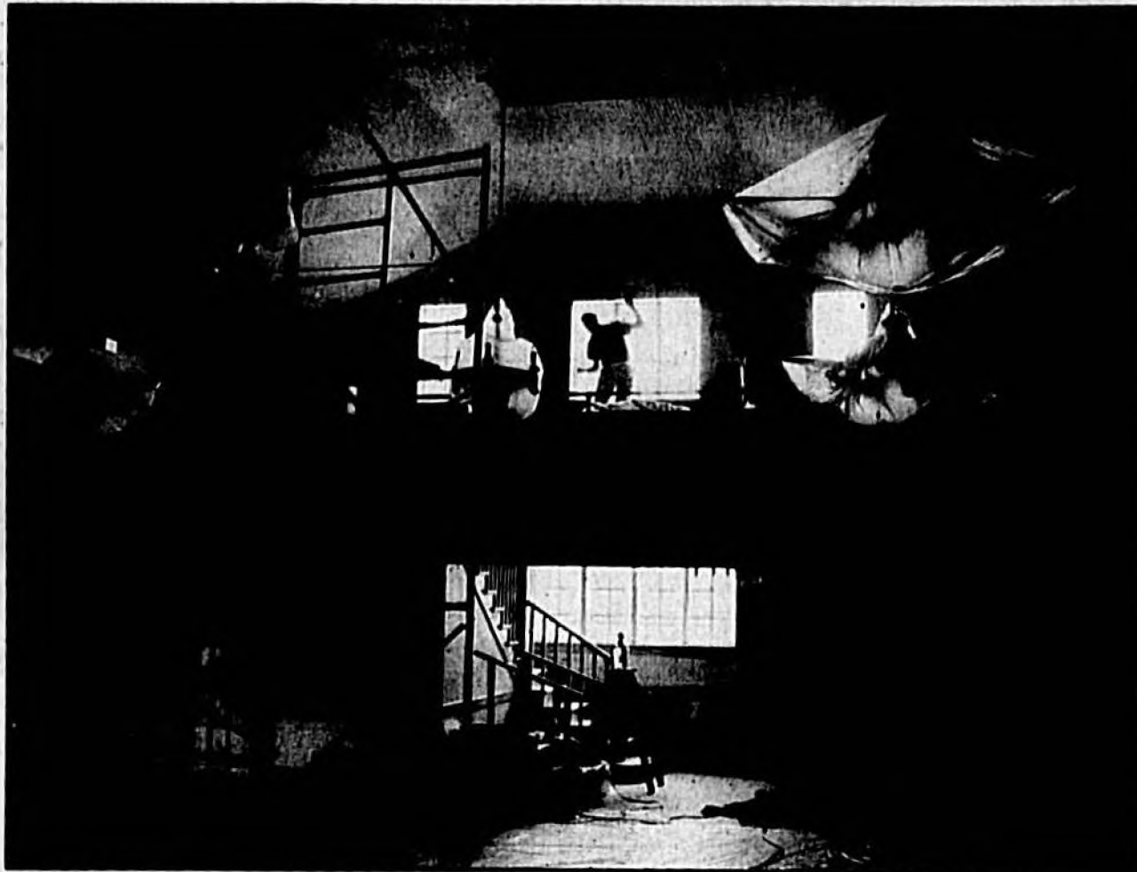
The Women's Club of Sanford is celebrating its 90th birthday this year. Recently, the club's building received a little TLC from Home Elegant Painting and Repairs. Steve, Barry and Brian Porter from the company prepare the interior of the building for painting by covering chandeliers and taping windows to prevent over spray, etc.
