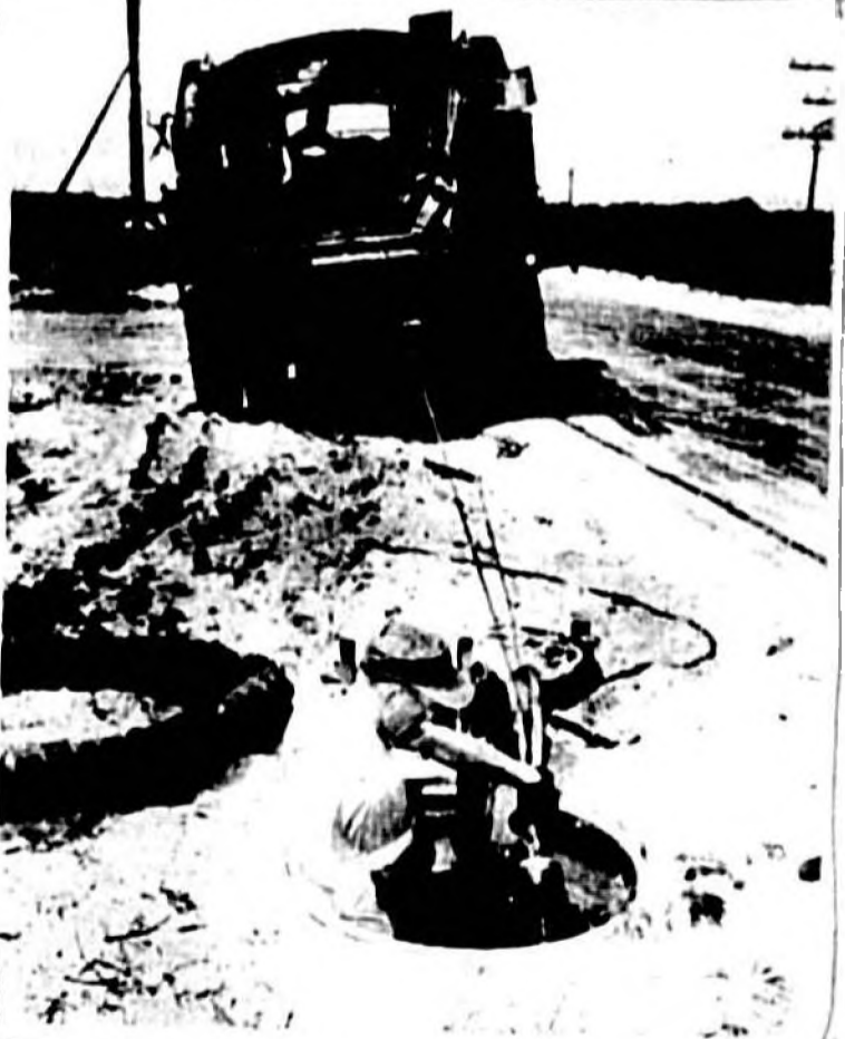
BECAUSE OF THE high winds that sometimes beset the area south of West Palm Beach, the Bell Company has taken its tower communications system underground for the 60 odd mile stretch to Miami. Here, workmen are placing one of the more than 600,000 feet of cable needed to complete the new system.
