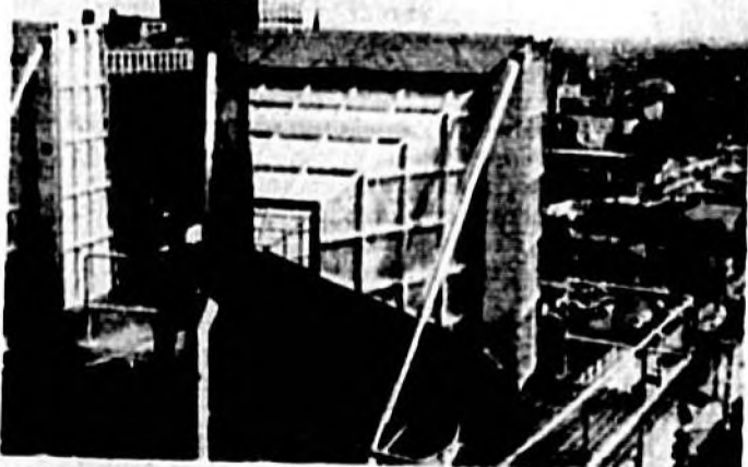
LOOKING LIKE something from outer space, this giant horn is one of a series extending from Jacksonville to West Palm Beach to "catch" thousands of long distance phone calls out of the air and relay them simultaneously along their route.
