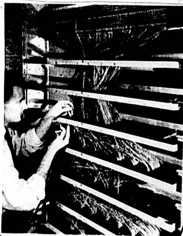
BELIEVE IT OR NOT! But this intricate maze of wires is only part of the equipment needed so that Bell Telephone Company can record charges on long distance calls made by Florida subscribers. This electrical "directory" converts an equipment number into a subscriber's telephone number, so that proper charges can be made.
