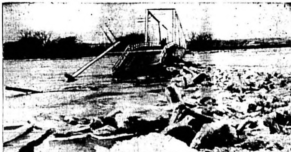
Ice on the raging Platte River, battered out a span of this bridge on the highway between Valley and Lehigh, Nebraska. These towns were with it gas when a pipe line attached to the bridge snapped as the span was washed out. (Associated Press Photo)
