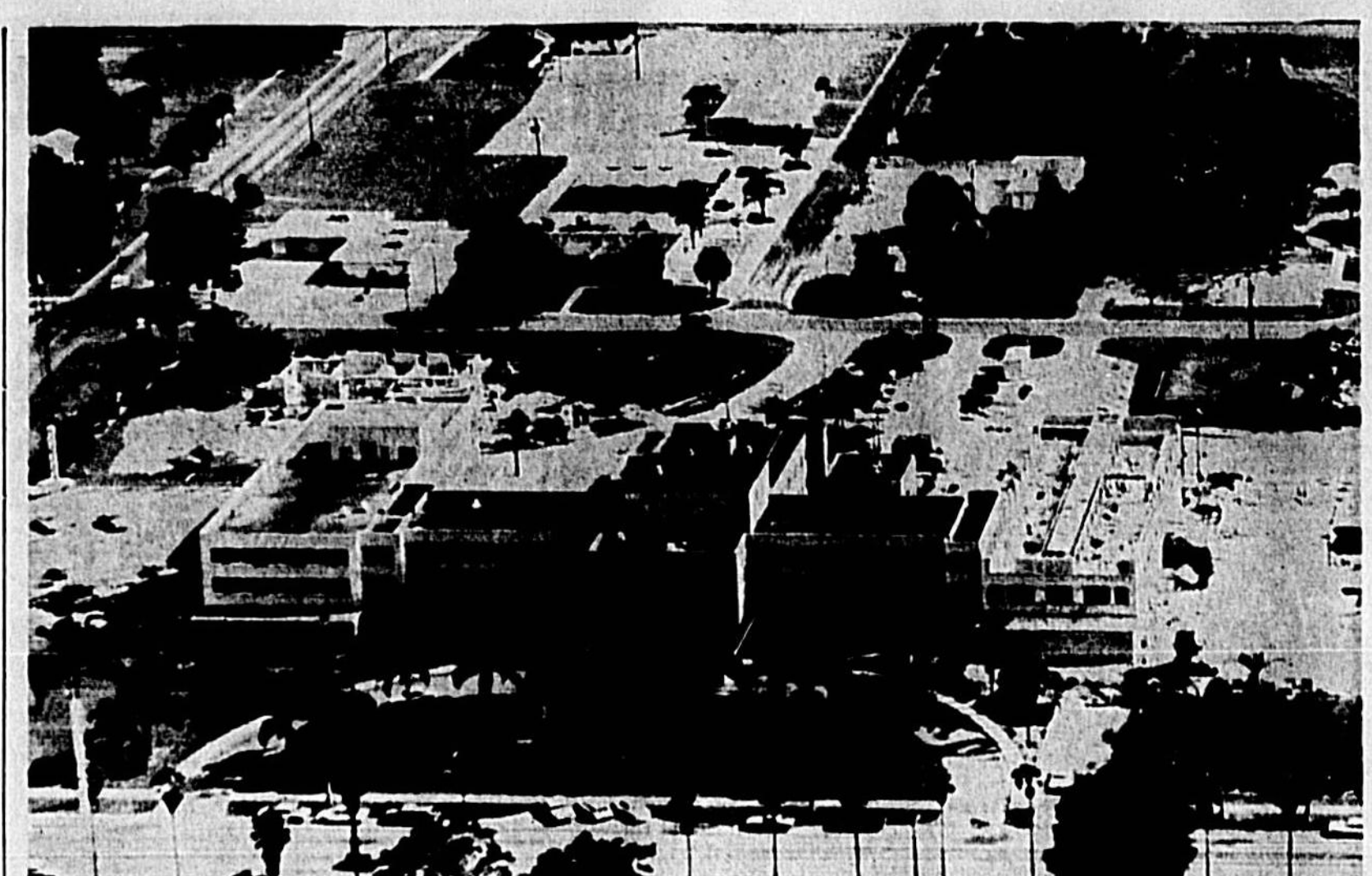
MILLION-DOLLAR wing of Seminoles Memorial Hospital is going up! Progress of the facility is pictured at the right of the present plan. New boiler room is at the left rear of the hospital. Administrator Robert Besserer said today the new wing will be placed in operation in March or April. (Aerial photo by Herald photographer Bill Vincent Jr. from a flying Seminoles Ranch airplane.)
