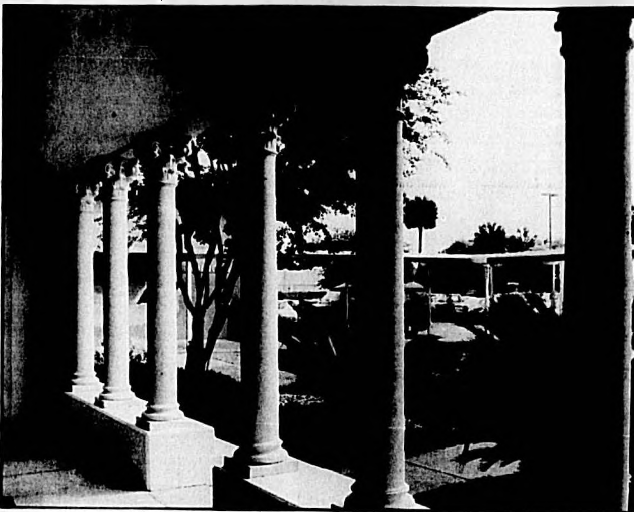
These ornate columns at Sanford Middle School are used as support columns for the front of the administration office. They were carefully removed from the old building that was demolished several years ago to make way for a larger middle school. The old school housed a high school and then a junior high school before being replaced with the new existing middle school.
