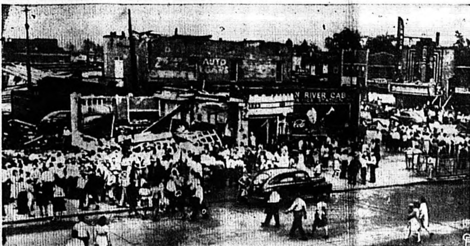
Crowds mill about in the business section of River Rouge on the outskirts of Detroit after a tornado struck the city by surprise, killing seventeen persons and injuring over 200 others. At right, a motion picture theatre stands badly damaged while in the foreground a crowd has gathered about a service station that has been completely ripped apart by the fury of freak storm.
