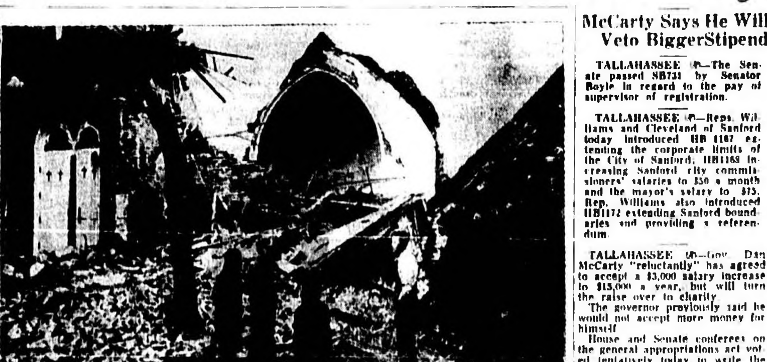
A mural of Christ stands out in the wreckage of the Sacred Heart Catholic Church at Hebron, N.C., after a tornado. The church, a three-story building, was destroyed; the altar and mural untouched. Stones were injured and damage was estimated at $1,500,000. (AP Wirephoto)
