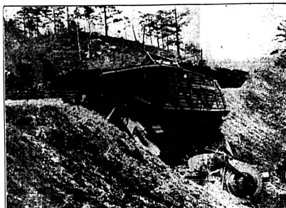
Two trainmen, brakeman J. M. Brown and fireman Frank Kenamer, were killed near Maxwell, Ala., in the wreck of a freight train caused by flood water. The locomotive, which can be seen buried in the ravine, and a number of cars plunged from the track undermined by the torrents. (Associated Press Photo)
