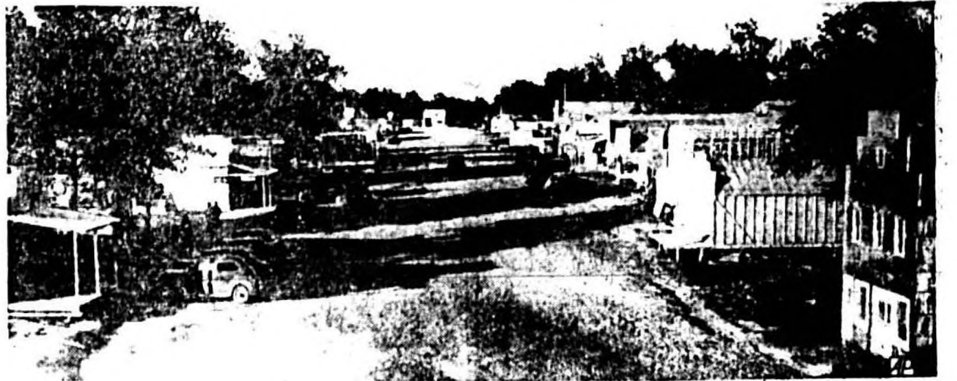
BOOM DAYS IN DISNEY, OKLA. haven't ignited the town's Main street yet (above), but wait and see—says this community springing up beside federal $20,000,000 Grand River dam project.
