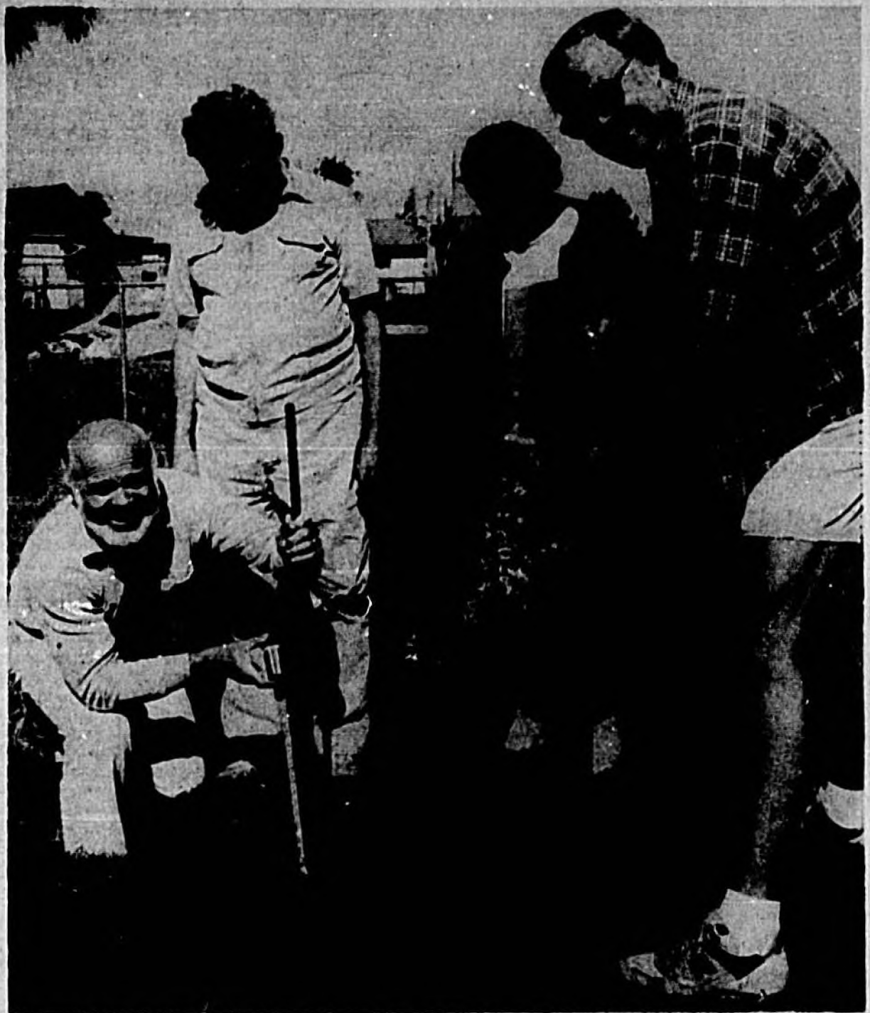
Don Nolt, (l) stakes the ground for Habitat for Humanity's first home in Midway. Assisting are
