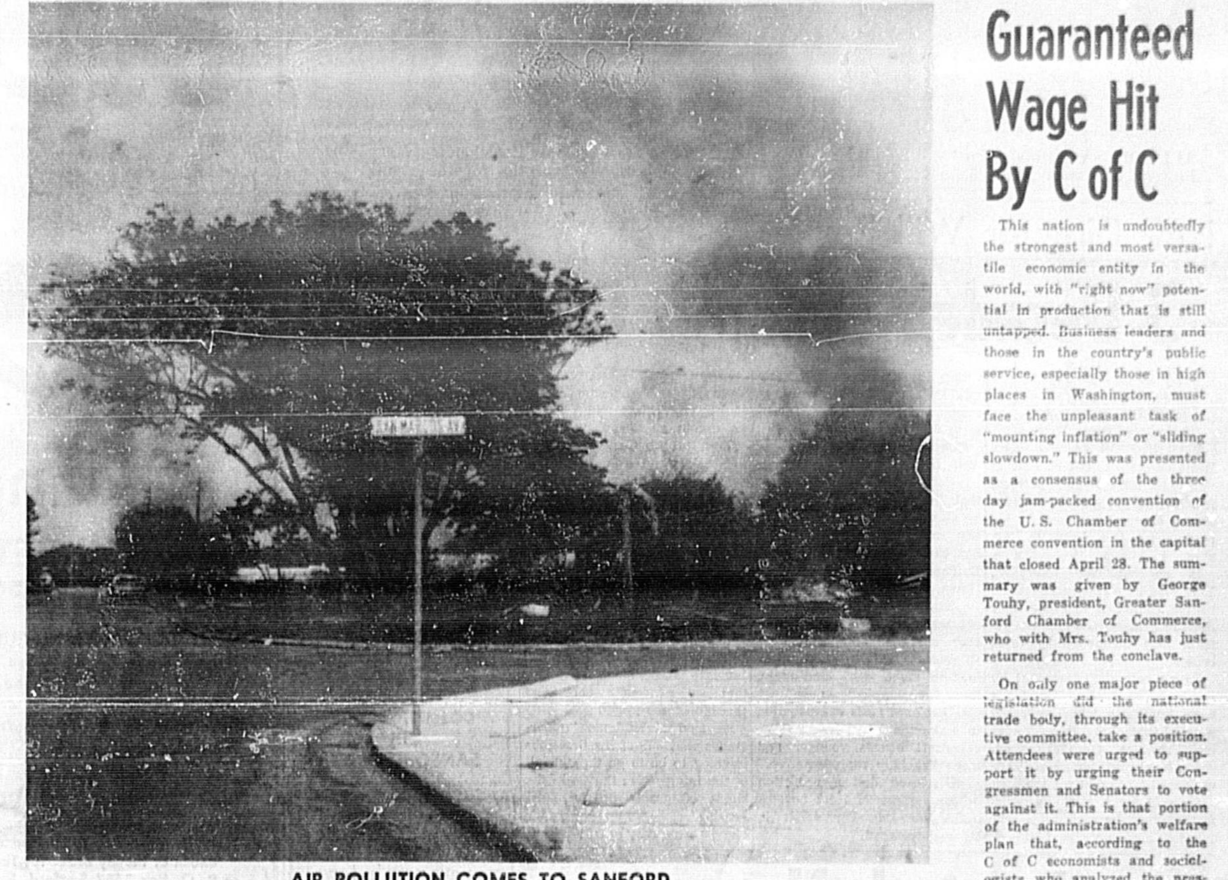
AIR POLLUTION COMES TO SANFORD SMOKE FILLED the sky in the vicinity of Seminole Memorial Hospital this morning as debris from the razing of a frame residence was burned.
