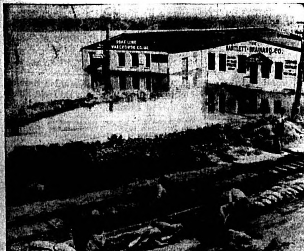
Workers at Hartford, Conn., where the rapidly rising Connecticut river brought new threat of food disaster, pitched in with a will and worked day and night throwing up sandbag dikes against the spreading flood waters. Part of a crew is shown at work along a railroad that parallels the river.
