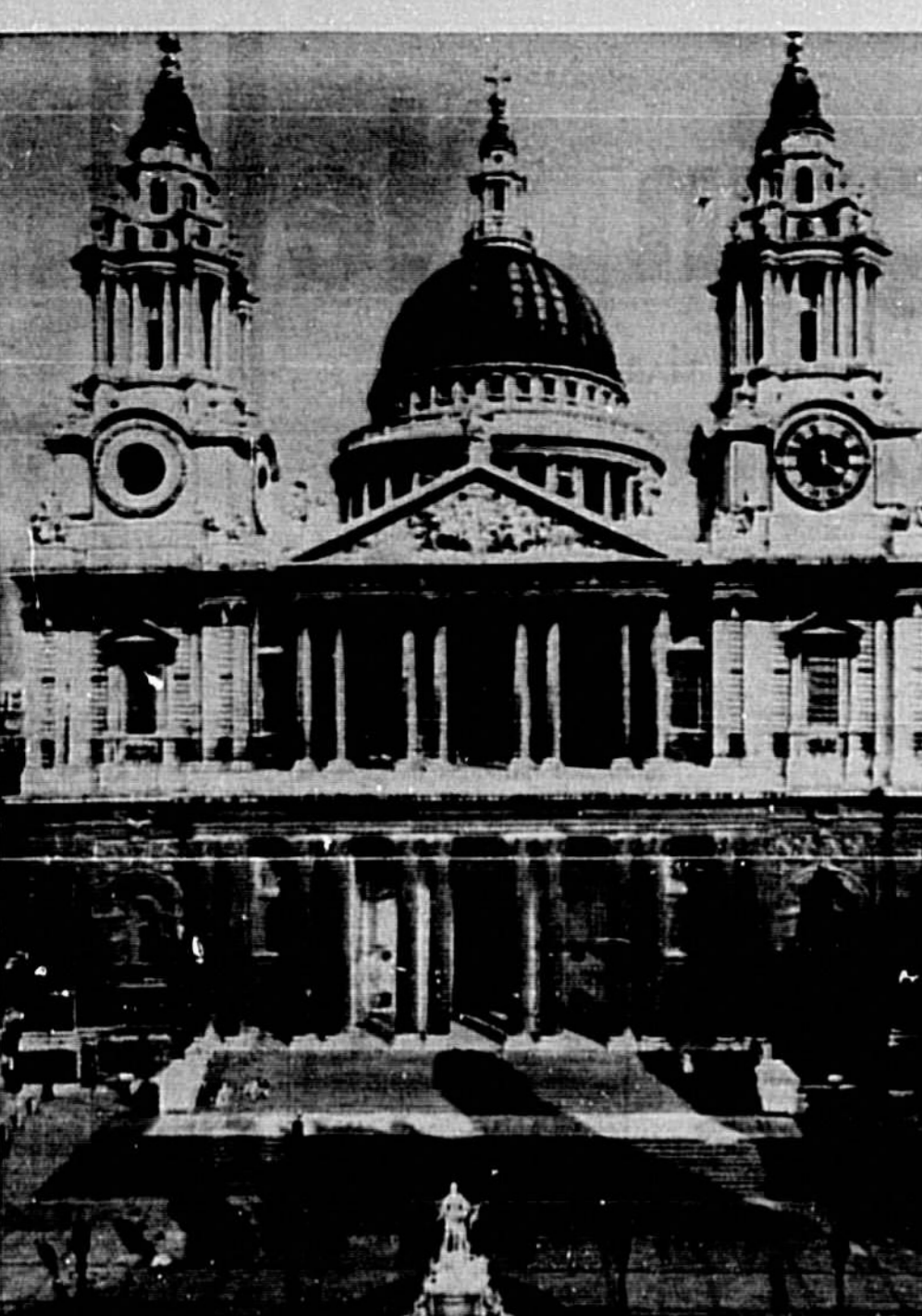
THREATENED — Portions of St. Paul's Cathedral in London may have to be closed to the public because of damage done by World War II German bombs and general deterioration. Cracks were discovered in building when it was cleaned about four years ago.
