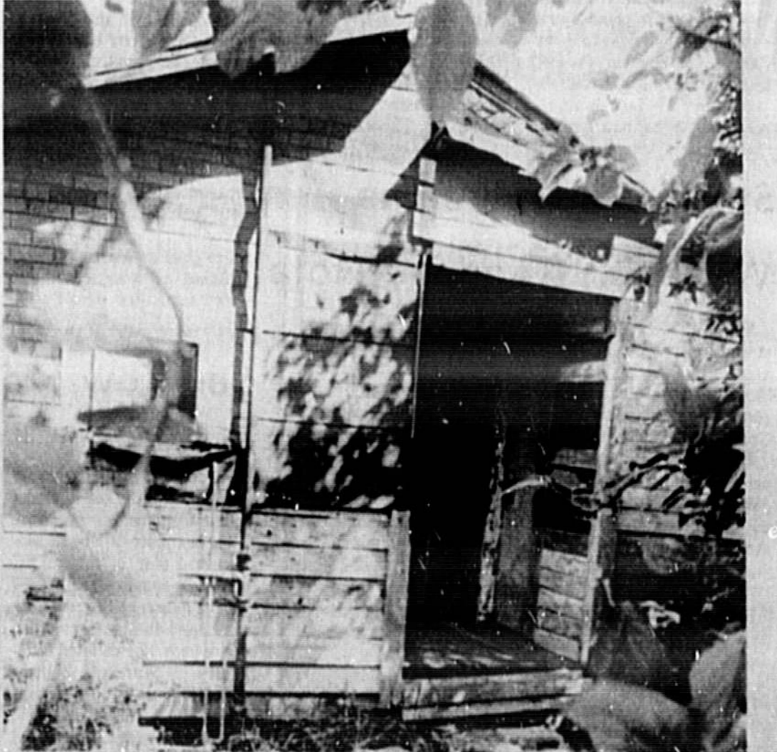
REAR SEALS BROKEN BY INTRUDER Day after investigators searched house
