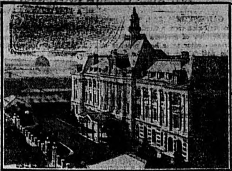
The State Capitol at Yokohama, one of the biggest and most modern of buildings in Japan, is reported to have collapsed in the earthquake.
