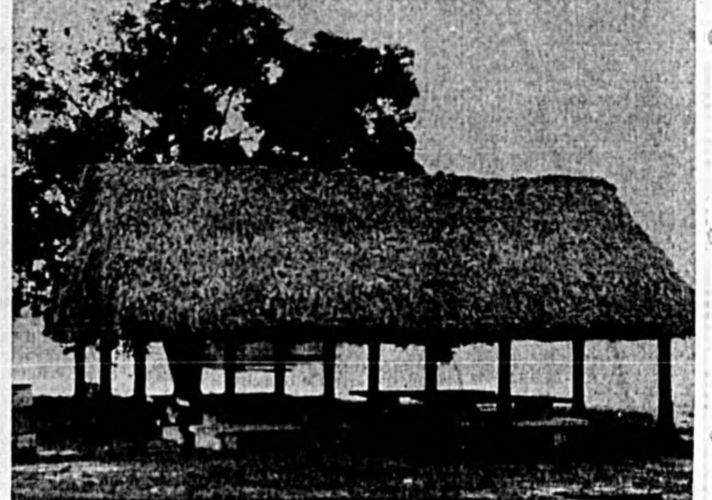
CRYSTAL LAKE picnic shelter stands idle on a cold day.
