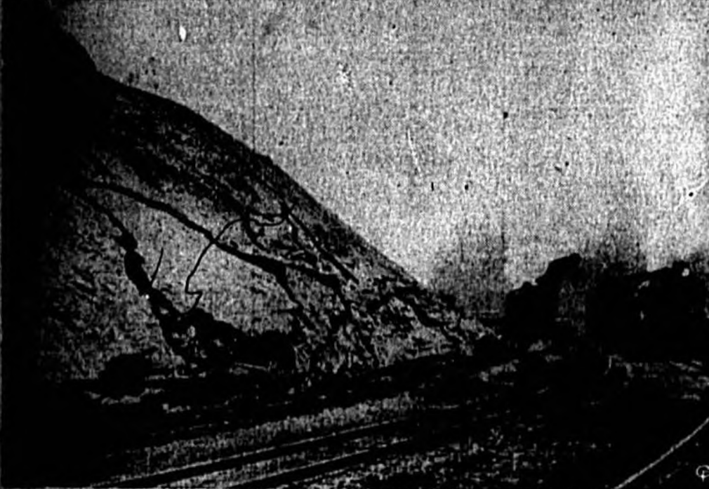
Railroad tracks are shoved aside, buckled and twisted out of shape as result of a landslide near Pittsburgh, Pa. An estimated million tons of dirt and rocks came down the hill to disrupt traffic on the Conemaugh Division of the Pennsylvania Railroad.
