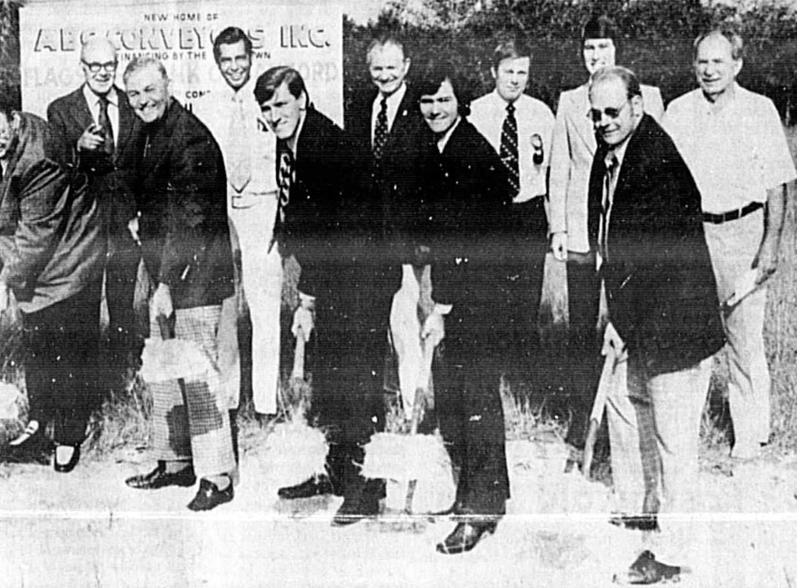
ABC CONVEYORS SHOVELS TURNED Another new industry broke ground this morning as ground breaking ceremonies were held for ABC Conveyors, formerly of Longwood, on South Sanford Ave. Helping get the construction of the 10,000 foot building to a start are, front row from left, Leroy Robb, contractor; Julian Stenstrom, city commissioner; Mayor Lee Moore; Cliff Wolfe, vice president of ABC; Brad Hollingsworth, Flagship Bank Downtown; and Donald Keen, president of ABC. Back row from left, Cliff McKibbin, Sanford Chamber of Commerce; Garnett White, Chamber of Commerce; Scott Burns, Chamber of Commerce and Florida Power and Light; Ken Barbaugh, FPL Community relations; Jim Whaley, Flagship Bank Downtown; and John Krieger, Chamber of Commerce. The new plant will cost $100,000 and will employ 35 to 50 people, which is expected within 90 days.
