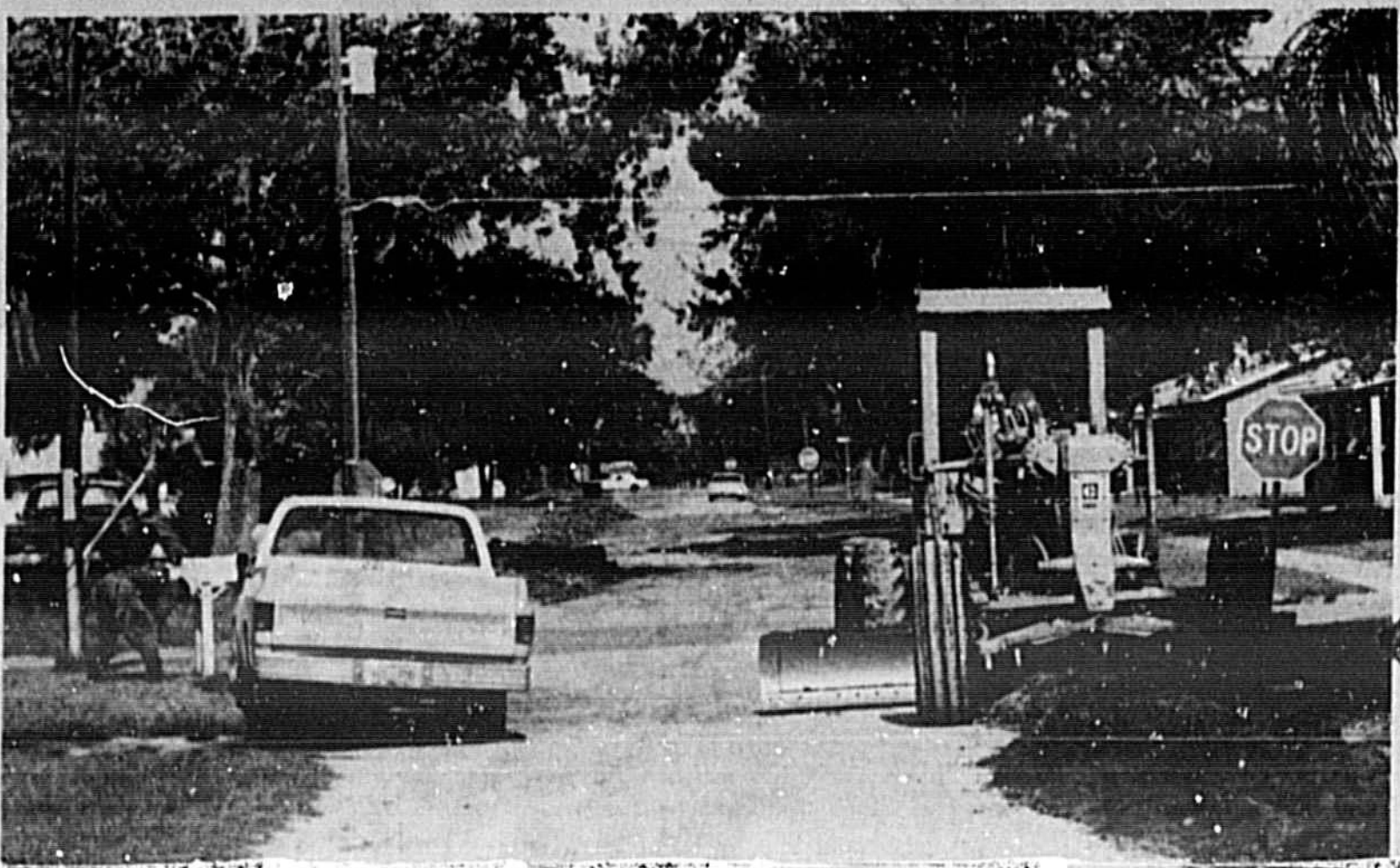
Sanford paving project gets underway at Fourth and Oleander Ave.
