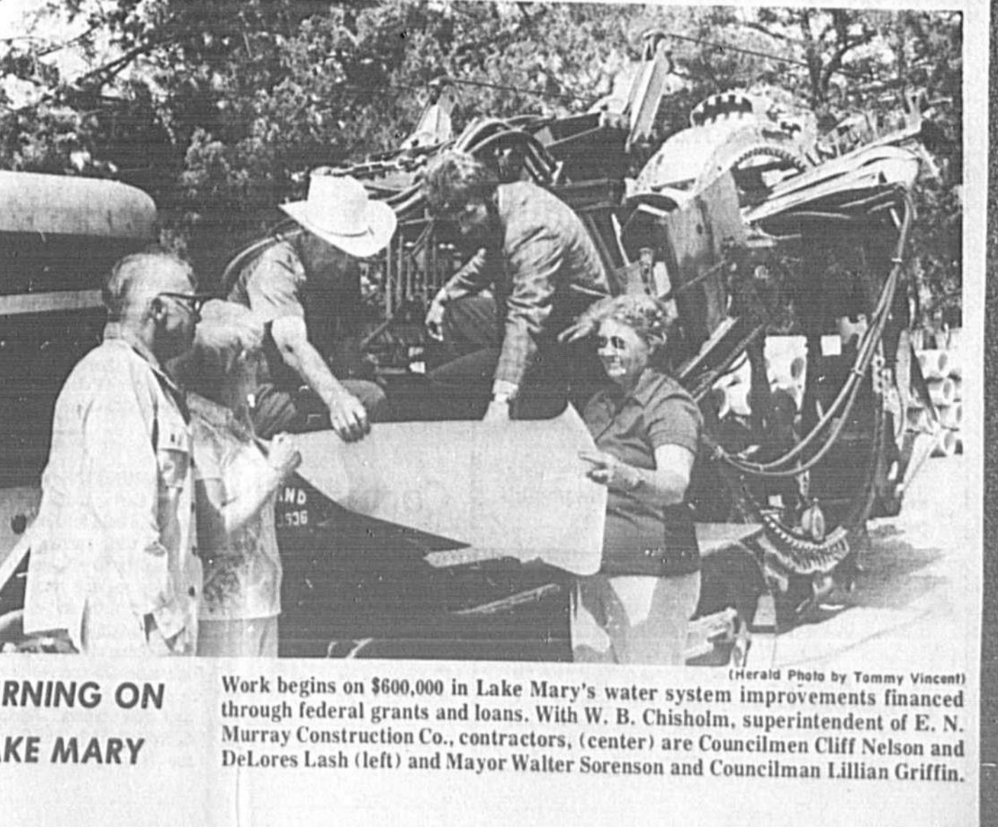
TURNING ON LAKE MARY Work begins on $600,000 in Lake Mary's water system improvements financed through federal grants and loans. With W. B. Chisholm, superintendent of E. N. Murray Construction Co. contractors, (center) are Councilmen Cliff Nelson and DeLores Lash (left) and Mayor Walter Sorenson and Councilman Lillian Griffin.
