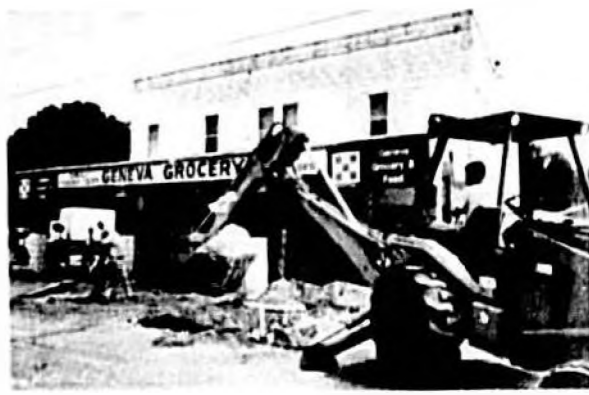
Excavation yesterday at Geneva Grocery.
