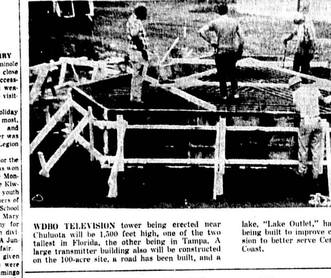
WHICH TELEVISION tower being erected near Chulutha will be 1,500 feet high, one of the tallest in Florida, the other being in Tampa.
