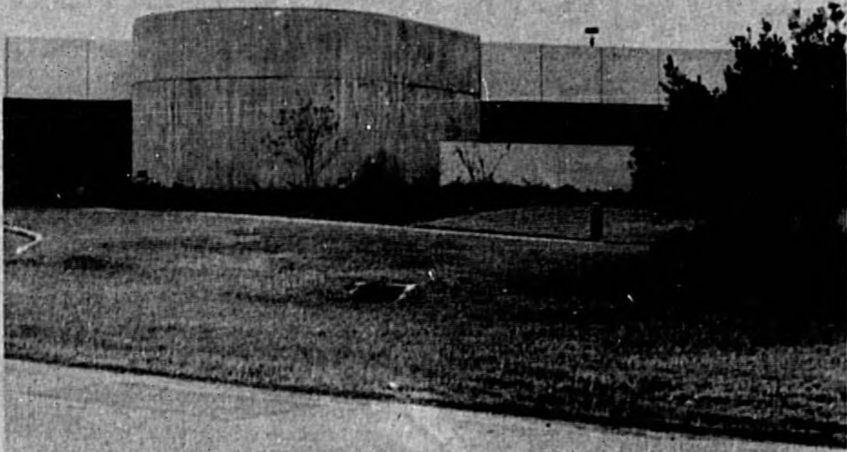
Walls of concrete house a linear accelerator heart of Central Florida Radiation Therapy Associates, on 200 Mangouline Ave., behind
