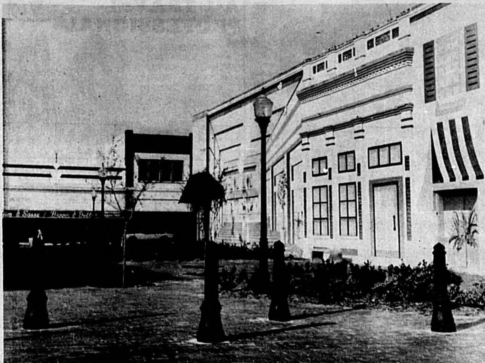
The brick-paved Magnolia pedestrian Mall is one of the highlights of Sanford's downtown redevelopment. The first block of Magnolia Avenue, south of First Street, is closed to
