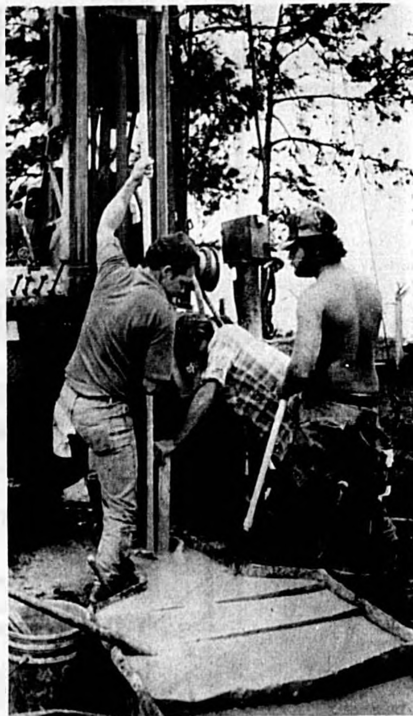
A Test well is drilled at Sanford's new well field off Oregon Avenue. Faced with a water shortage after EDB contamination was found in city wells at the Mayfair golf course, the city, in addition to rehabilitating the wells there, drilled four new wells at Hidden Lake park and purchased the new well field for future expansion.
