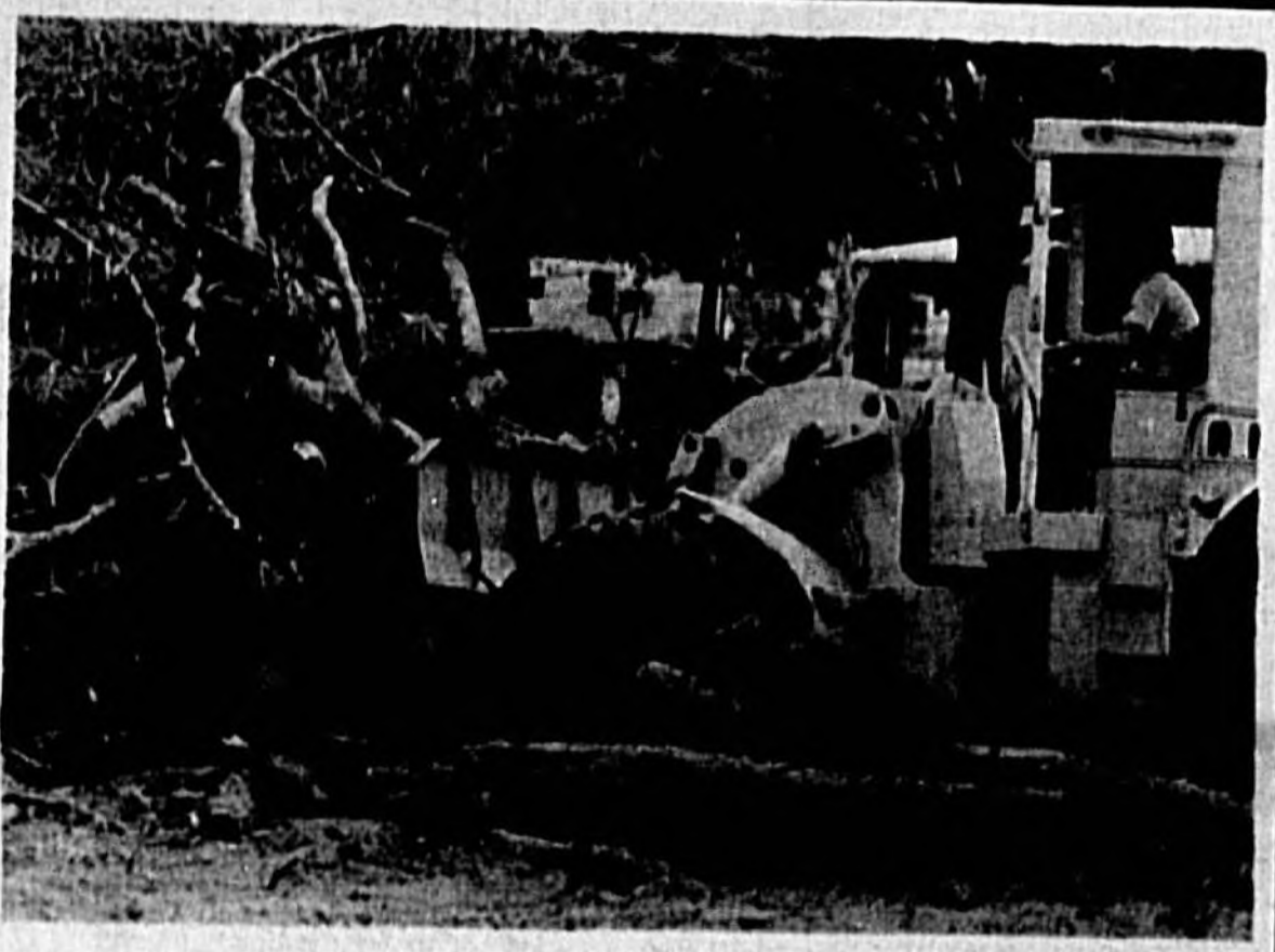
Junior Simmons of Fields Land Clearing Co. uses a front end loader to push a pile of cut pine trees at the Altamonte Library, 291 Mailland Ave. The trees were removed to make room for library expansion. Herald Photo by Gregory Gehret
