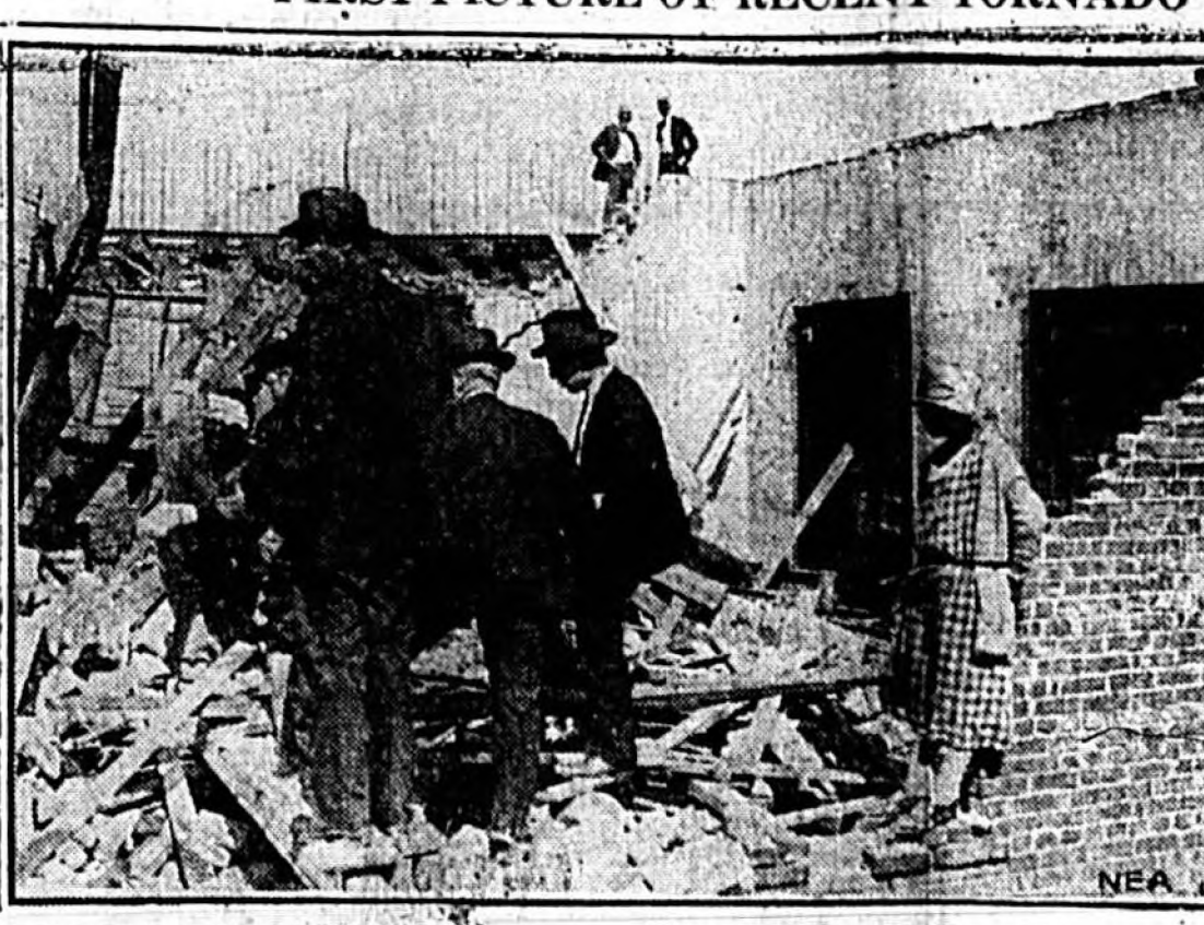
Just one of the many buildings which were demolished when the tornado swept through Georgia. This is the office building of the A. T. Small Co. at Macon, Ga. Eugene Threat (negro) with bandaged head was one of many buried under debris of the building.
