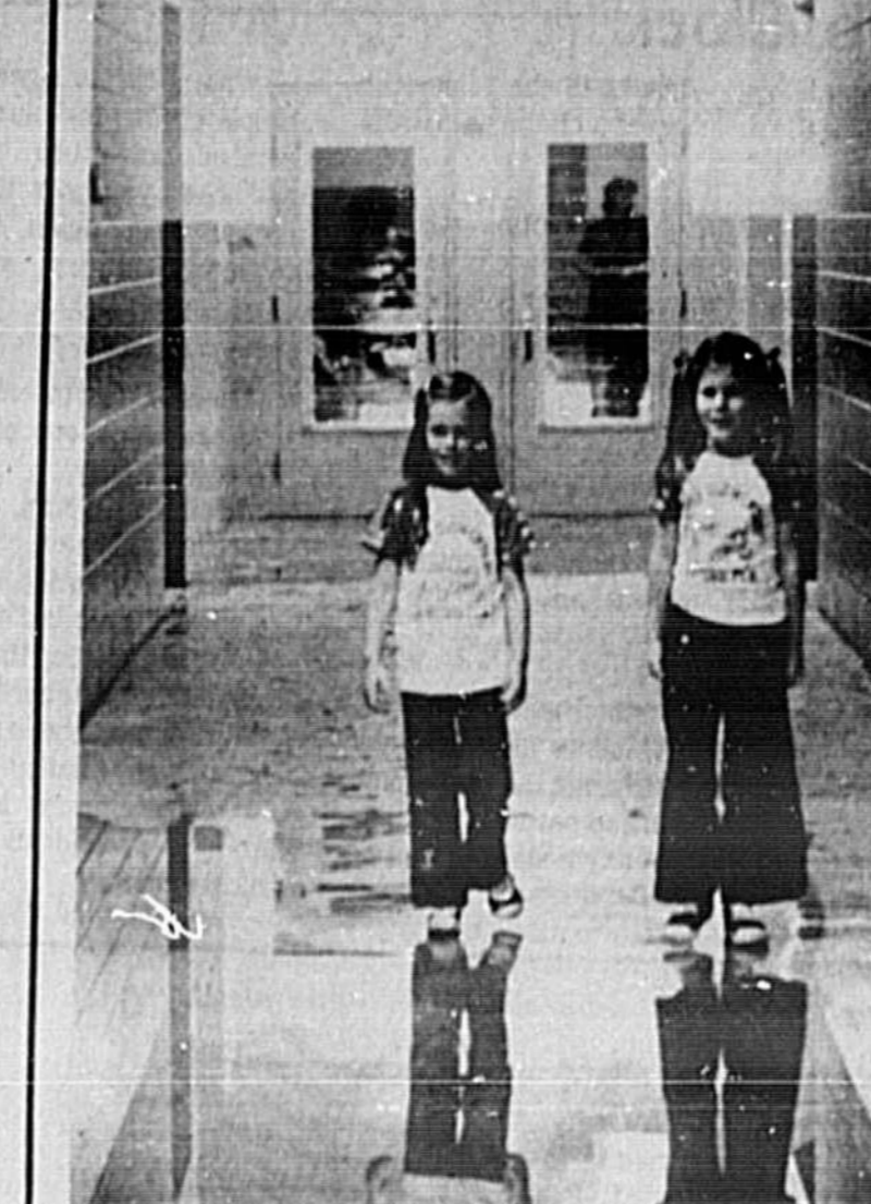
FLOODED SCHOOL CORRIDOR
