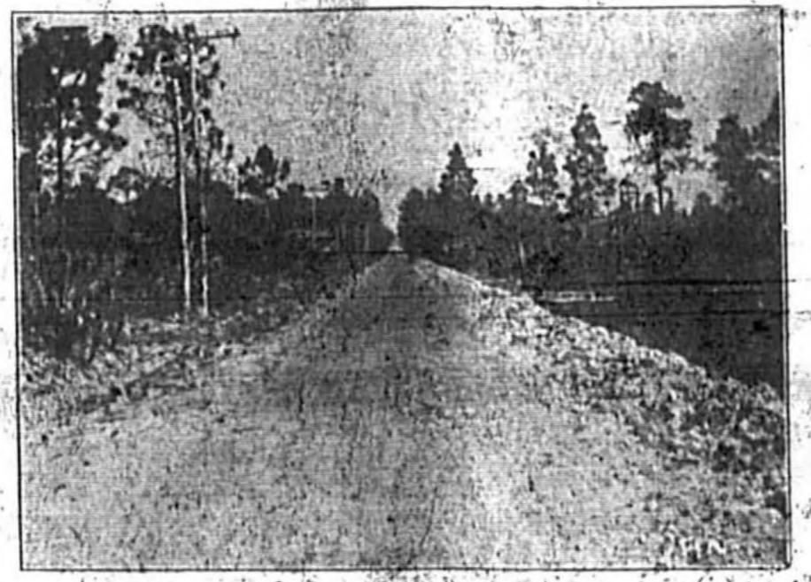
CUT SHOWS NEW BRICK ROAD NOW BEING BUILT SOUTH OF SANFORD
