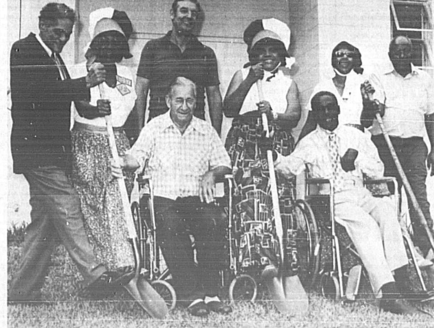
PATIO PROJECT Groundbreaking for the beautification and patio project at Good Samaritan Home was held Friday with home supporters and residents participating. Just Us Club is trying to raise funds to complete the patio to provide a place outdoors for residents to relax. From left, GSH Board member Dr. George Starker, Hilda Mitchell, vice president of the club; Jack Horwar, Greater Sanford Chamber of Commerce; Just Us President Mary Smith, Edna Field, secretary and Timothy Wilson, business manager for the home. In wheelchairs are Irvin Morris (left) and James Holmes.
