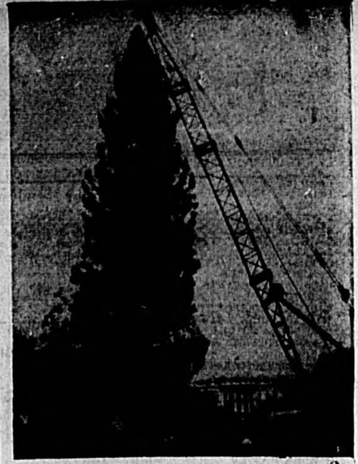
PREPARE FOR CHRISTMAS PAGEANT—A crane places a huge Christmas tree on the Ellipse near the White House in Washington. The 60-foot Minnesota white spruce will be the centerpiece of the capital's annual Christmas Pageant of Peace. (International)
