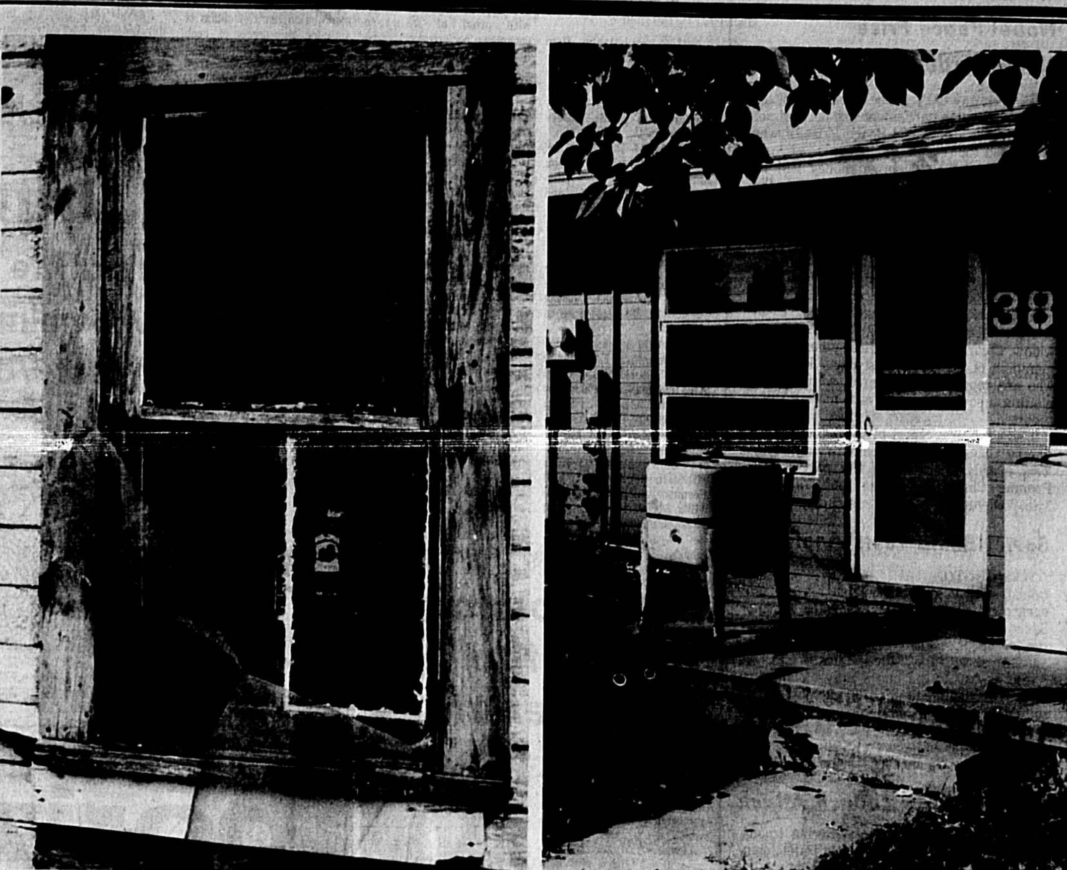
BAY AVE. KITCHEN WINDOW: THE WAY IT WAS
