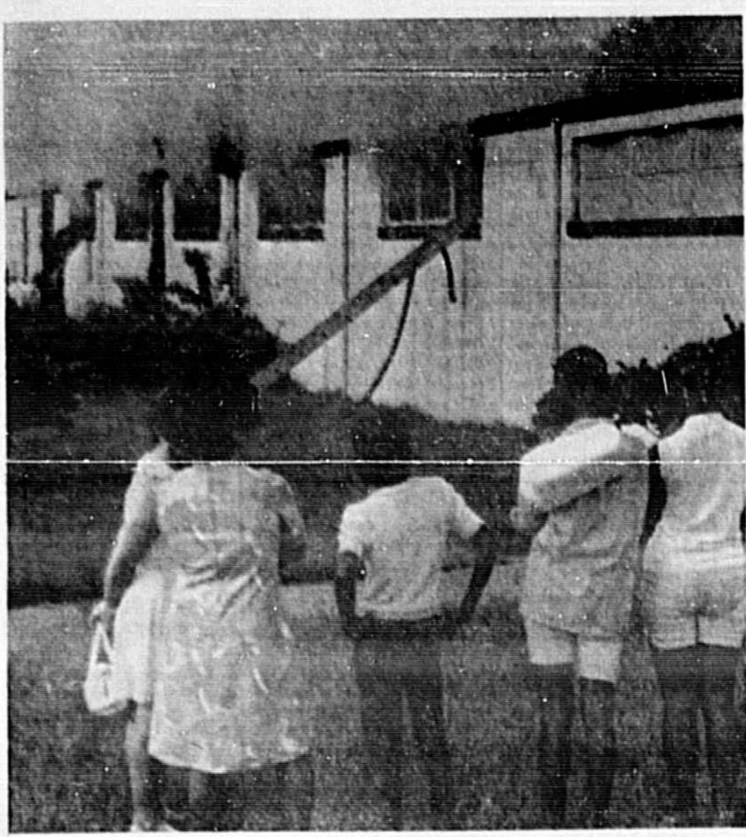
BYSTANDERS and employes watched Sanford firemen yesterday afternoon as they battled to control a blaze which razed Sanford Manufacturing. The firemen fought the blaze for over three hours before bringing it under control. Related photo on Page 1A. (Don Vincent Photo)
