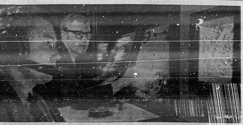
AIRCRAFT PATHS by the dezens build up on display screen of new computer said to be solution to until traffic jams. Goodyear computer reportedly is capable of sorting out those planes on a potential collision course and showing them on screen by themselves as an aid to air traffic controllers.
