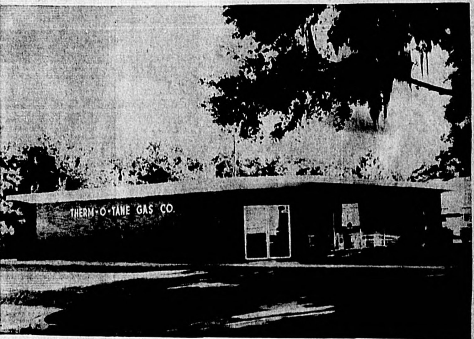
THERM-O-TANE GAS & APPLIANCE CO.'s office, showrooms, and warehouse where formal opening is being held tomorrow. A large parking lot for customers is located on the Laurel Ave. side of the building located at 414 W. 9th St. (Photo by Jameson)
