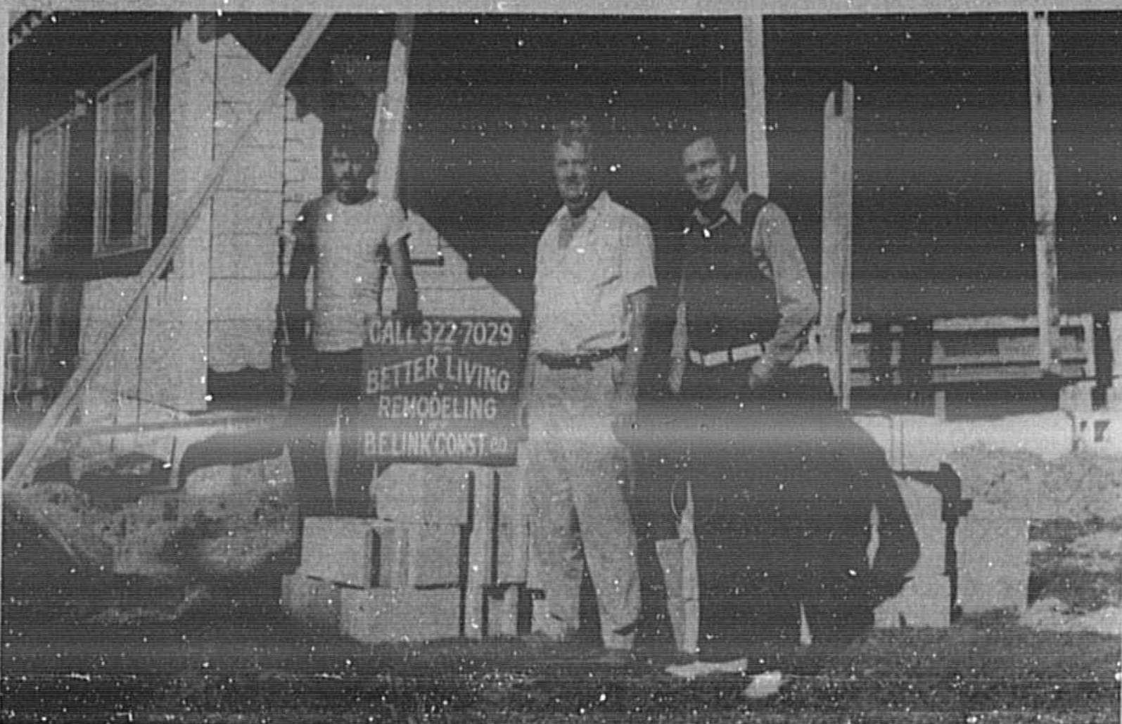
CONSTRUCTION TEAM REMODELS HOME (l to r) James Zavrotvy, B.E. Link, George Dillard
