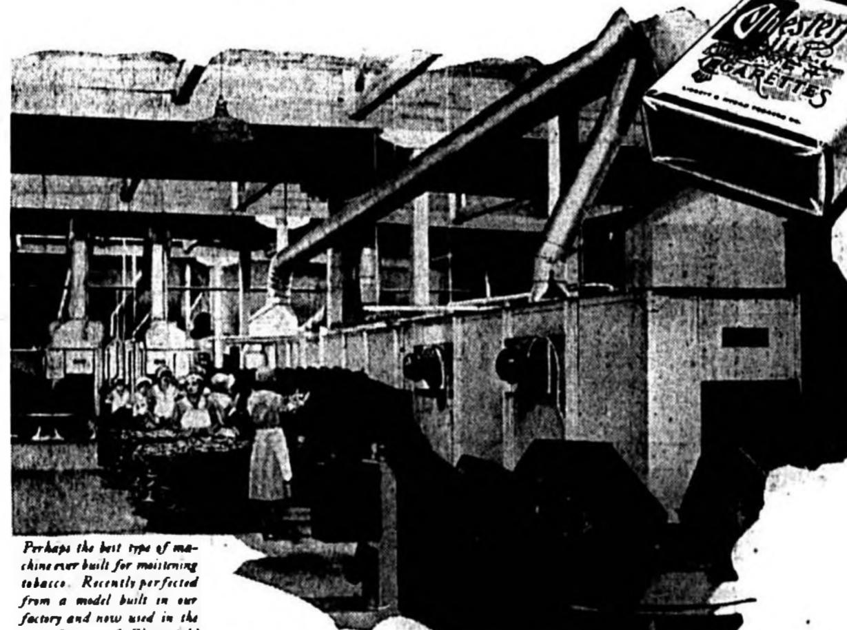
This picture shows the machine used to remove the stems from Chesterfield tobacco.
