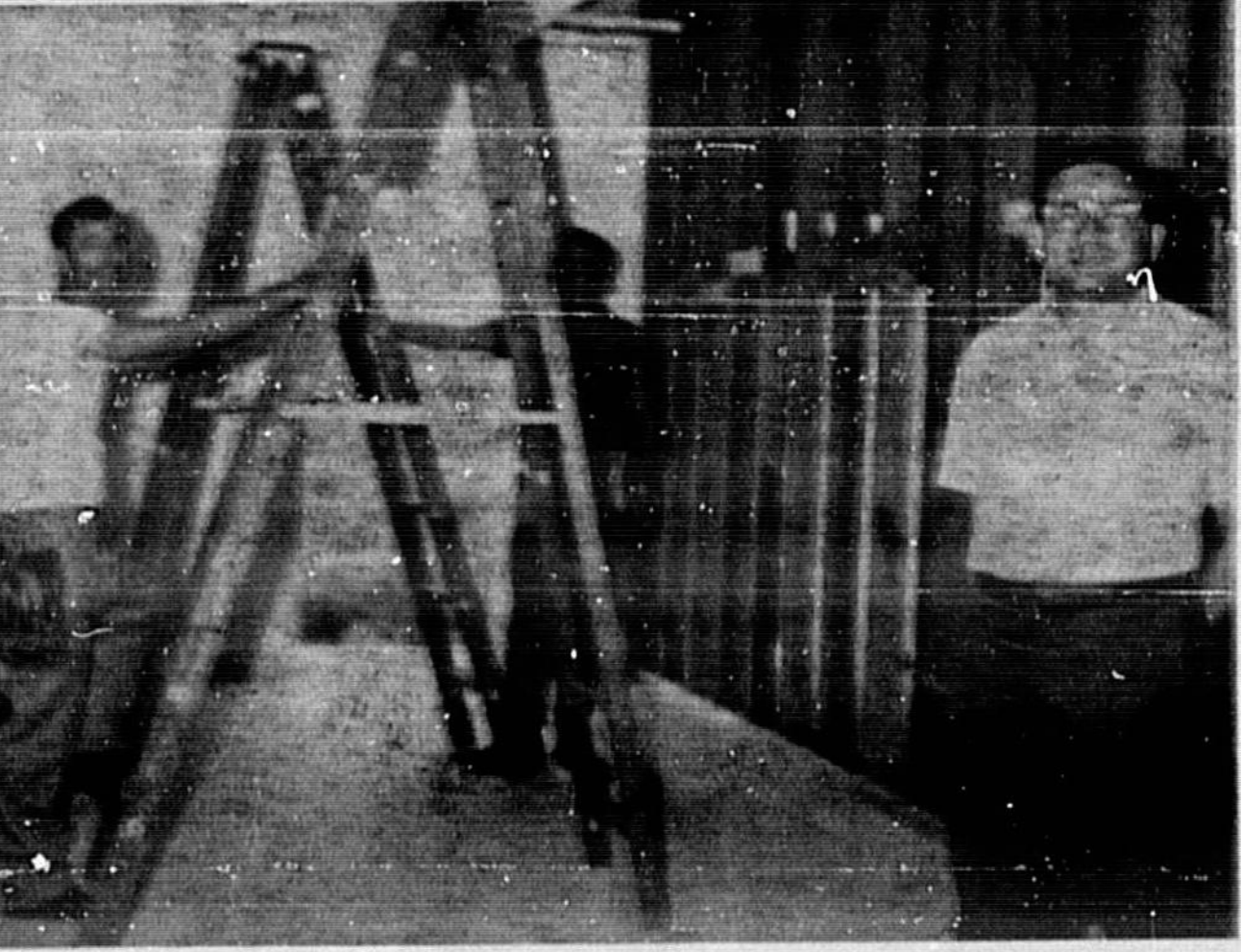
JUAN FALCON, owner and operator of FALCON & SON AIR CONDITIONING, HEATING AND REFRIGERATION oversees the construction in the office he will be moving into in less than two weeks. A big grand opening will be held December 15 at his new office. Try Juan "You won't be sorry."
