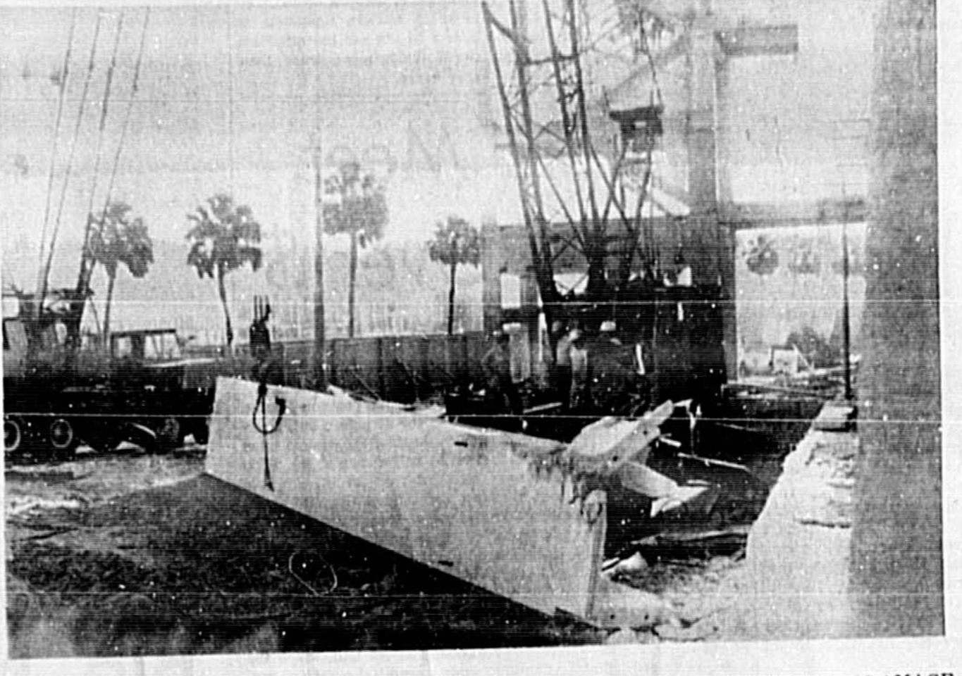
EXTENSIVE DAMAGE was done to a crane this morning on the construction site of the new county courthouse when a piece of exterior stone-work for the north wall fell (top photo) while being lifted into place. No one was injured in the mishap but the abutment and undercarriage of the crane was demolished (left photo). The exact amount of damage to the crane has yet to be determined. The architect for the courthouse, Richard Matz, said there was no damage of structural significance and construction is not expected to be delayed. The exterior work will resume when the replacement crane, which is expected today, arrives. (Bill Vincent Photos)
