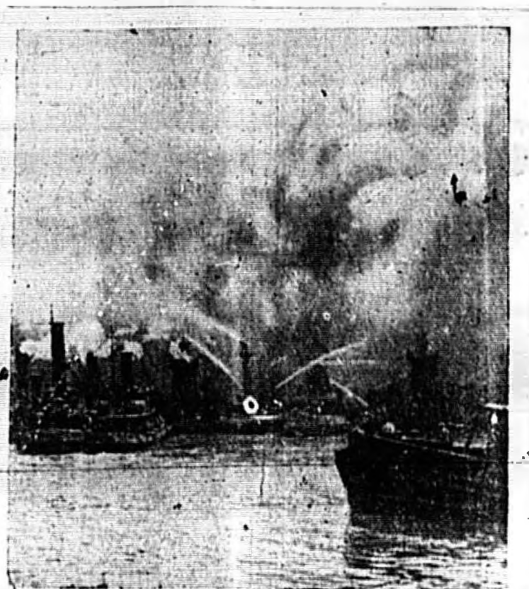
Streams of water are poured by fireboats on the flames raging through the Municipal Ferry Terminal Station Island, N. Y. Thousands of commuters between Manhattan and the island were temporarily stranded yesterday as firefighters sought to bring the conflagration under control. Two persons were said to have died in the fire.
