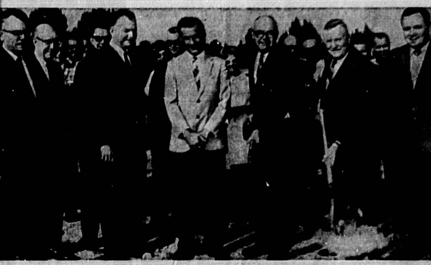
GROUNDBREAKING this morning at the site of the new Pinebreeze egg plant in Sanford Industrial Park on Sanford Avenue drew approximately 25 persons to watch Clifford McKibbin (left), president of Sanford-Seminole Development Company, and Bernard Johann, Pinebreeze president turn first shovels of dirt. Looking on are LeRoy Robb, project contractor, George Touhy, William Jarman, local plant manager, and Jesse Rowe, Pinebreeze vice president. (Herald Photo)
