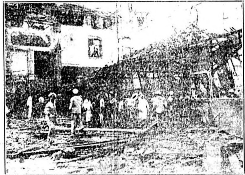
A view of the wreckage of one of the buildings at the Brazilian Naval Plant, just across the bay from Rio de Janeiro.
