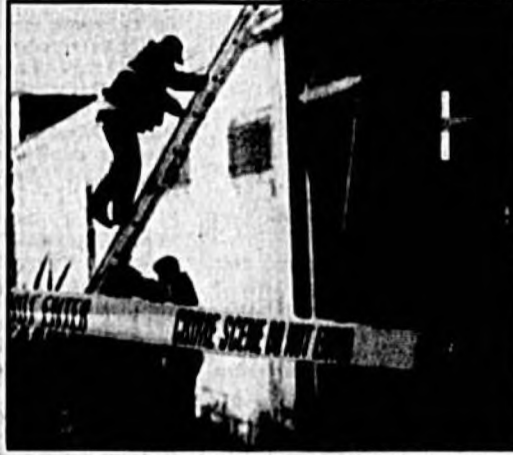
Herald photo by Tommy Vincent Investigators search the rooftop of the Sanford Masonic Lodge Wednesday with the help of the Sanford Fire Department in hopes of finding any clues that could break the recent wave of downtown burglaries.
